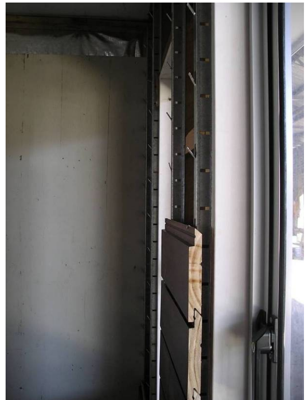
Photo 4: Side view of boards placed in between fins protruding from batten
