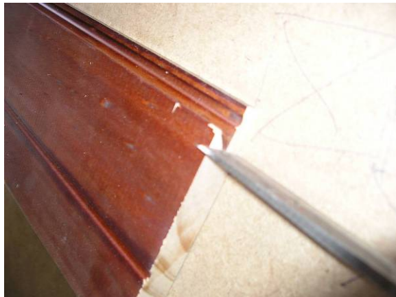
Photo 7: Connector (with adhesive applied) fitted behind board
