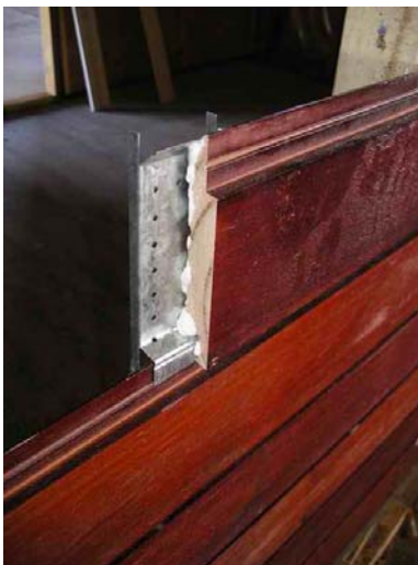
Photo 7: Connector (with adhesive applied) fitted behind board
