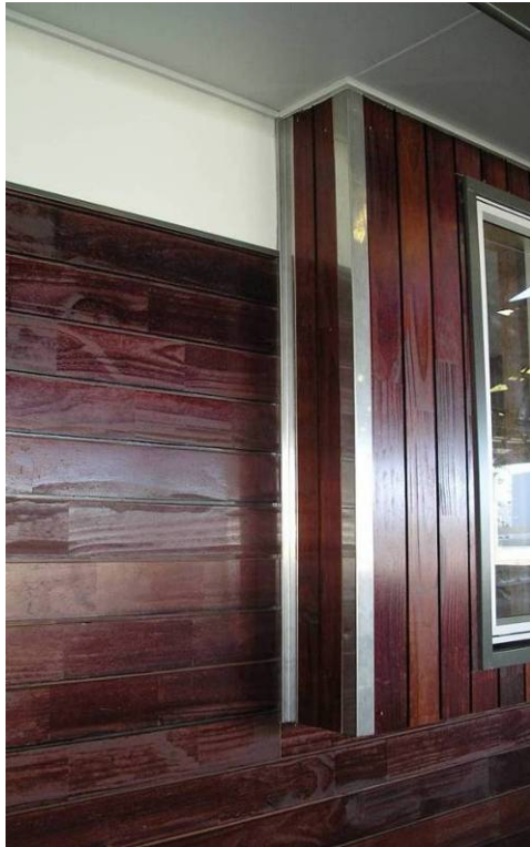
Photo 11: Example of stainless steel bent metal external and re-entrant corner flashings
