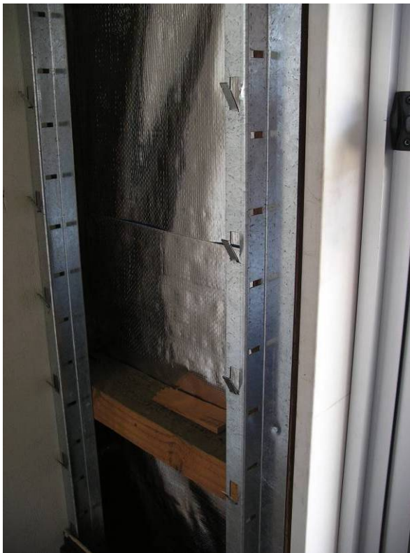
Photo 3: Metal battens fixed to the face of studs with fins protruding
