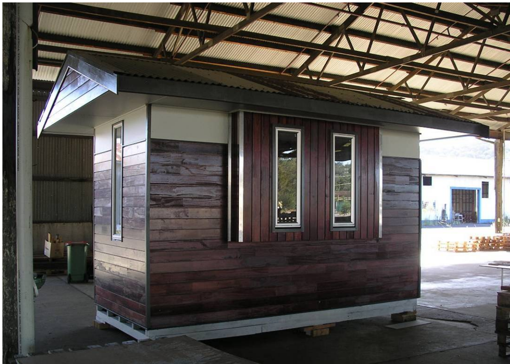
Photo 1: The Flatline prototype building
