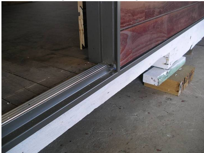
Photo 13: Cladding base (starter) flashing
