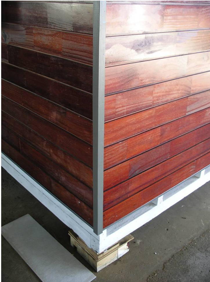
Photo 14: Perspective view of timber corner mould
